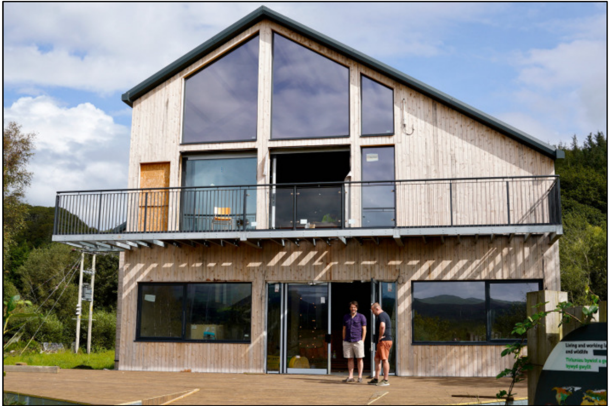
The Dyfi Wildlife Centre nearing completion
